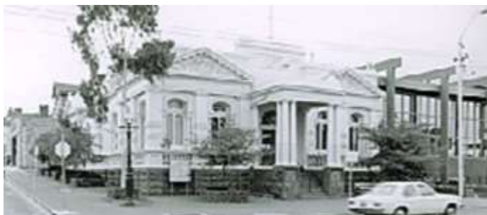
Free library (left), Municipal Offices (right)
